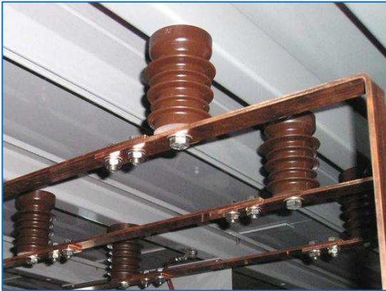
In our CP253 YY capacitor banks we propose bare copper bus-bars supported by epoxy type insulators.
