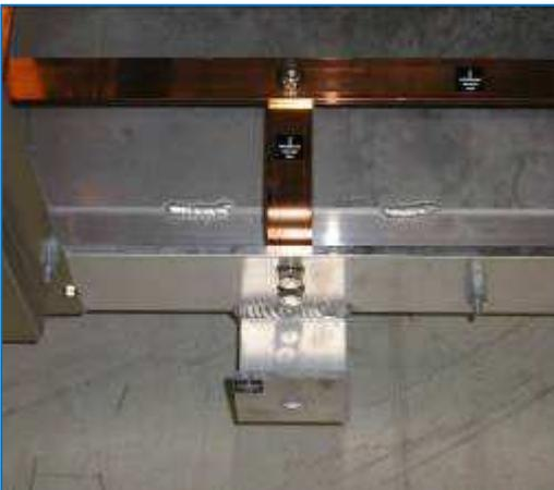
We use the capacitor bank aluminium chassis for grounding.
