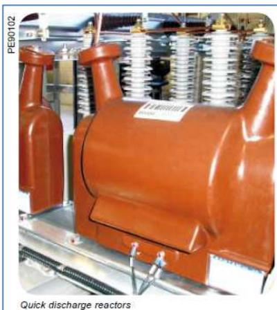
This option consists in having one set of 2 discharge coils per stage of the automatic capacitor banks
