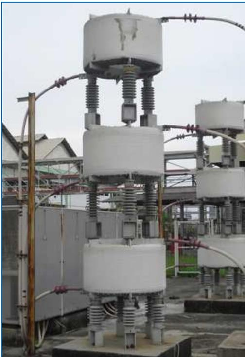
We can also provide “Single –phase, Air core type” reactors.
