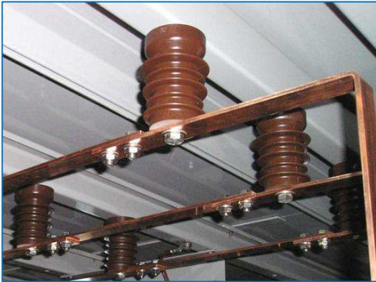
In our CP 253 YY SAH capacitor banks we propose bare copper busbars supported by epoxy type insulators.
